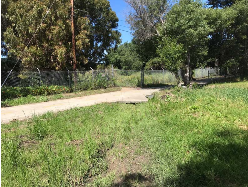
Photo 17. Drainage 1 crosses beneath bike path via small box culvert and flows onto Morro Bay Power Plant property. Due to vegetation growth along the channel to west, flows are impounded creating an area of seasonal ponding on the other side of the fence. See below photo.
